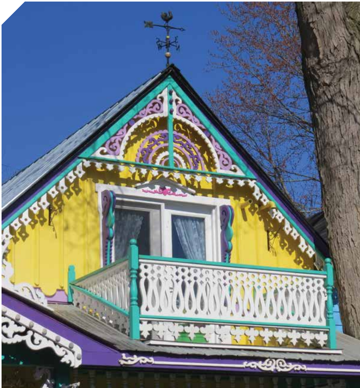
◀ The “sunburst” feature of gingerbread under the peak is common and found in both refurbished and historic houses.
